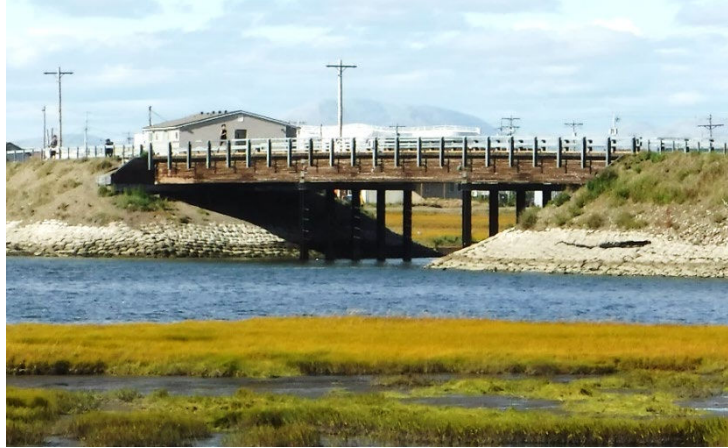
Ted Stevens Way Bridge over Kotzebue Slough, Bristol 2017
