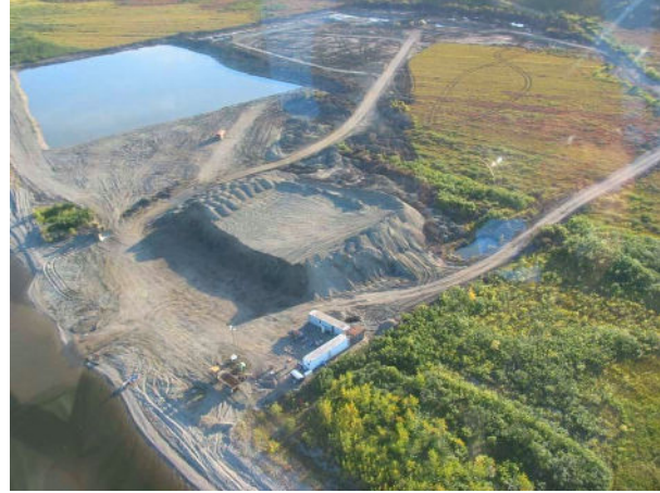
Gravel extraction at Nimiuk Point (Alaska DOT&PF)
