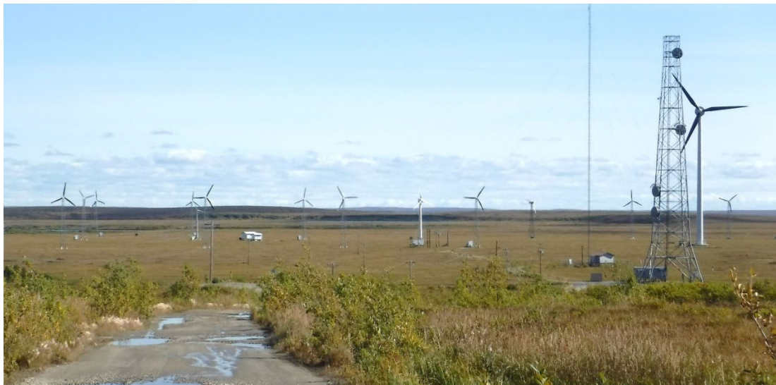
KEA Wind Farm off Kotz7 Road, Bristol 2017
